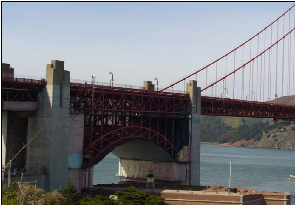
Photograph 7. Seismic retrofit in progress at Fort Point Arch, camera facing northwest, March 2007. [Source: JRP Historical Consulting, LLC]
