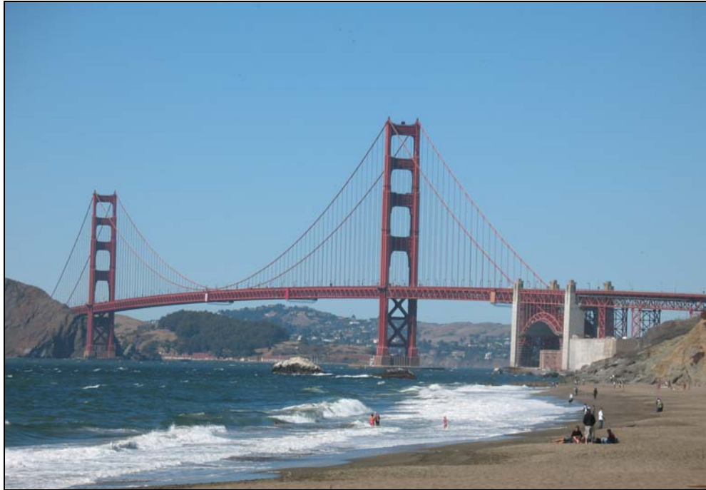
Photograph 3. View of west side of the bridge showing South Viaduct, camera facing northeast, August 2007. [Source: MacDonald Architects]
