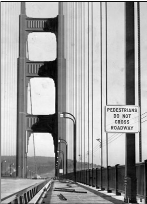
Figure 2. Photographs of sidewalk, railing, light standards and roadway. At left, just days before the bridge opened in May 1937, with original light fixtures. (San Francisco History Center, San Francisco Public Library) At right, showing replaced light fixtures, by photographer Jet Lowe, 1984. (HAER CA-31, www.loc.gov ). See Photograph 6, below for a view of the new public safety railing.
