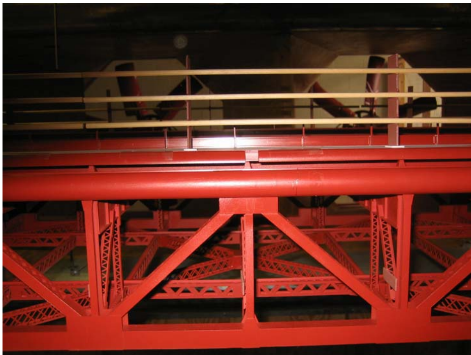
Vertical 12' barrier with wind fairings (Test number W1 Alt.)
